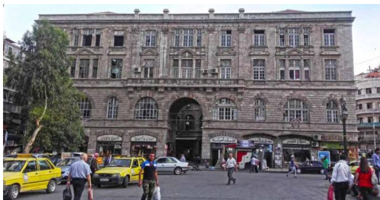
Fig. 9. A service building from the Ottoman period
